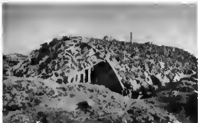
Figure 53. Here is a quonset hut blended into the terrain by a combination of digging in, texturing, and covering with a net.
